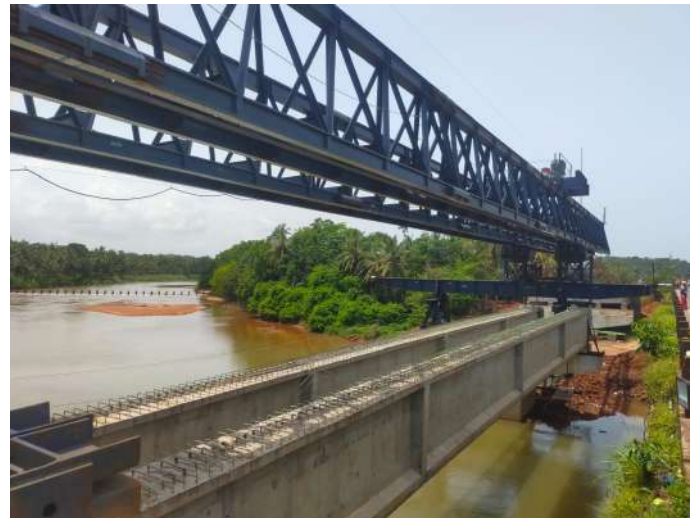
Section of Launching Gantry
