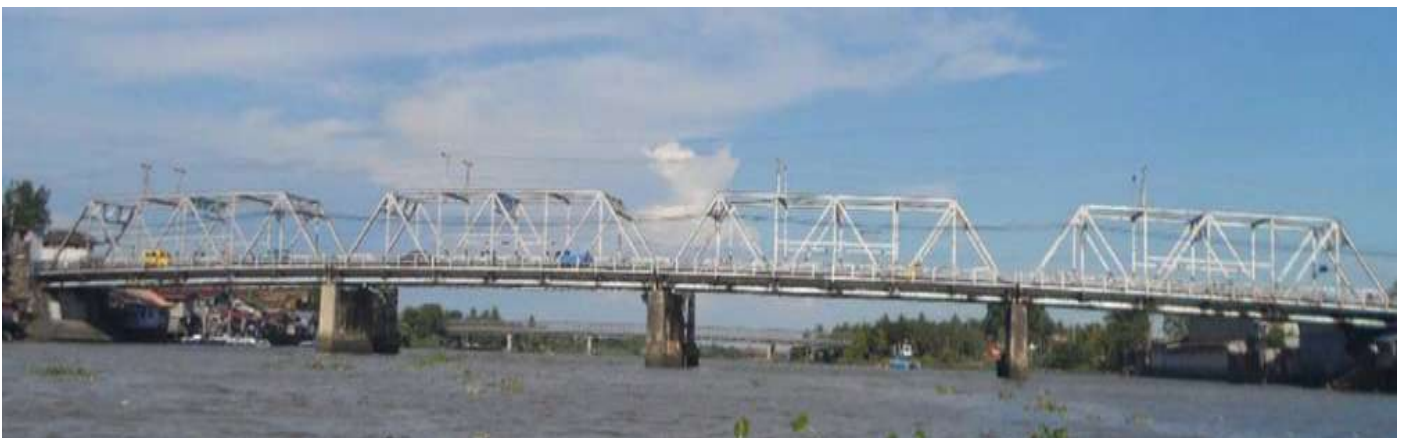
Typical Bridge Segment 40.25m
