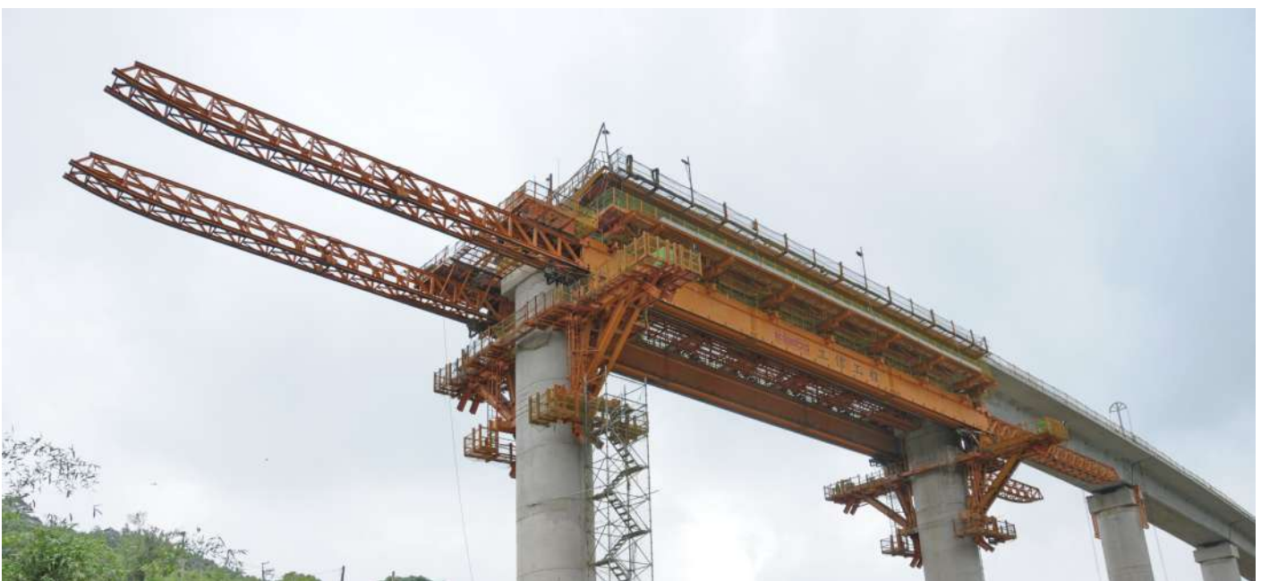
Typical Deck Inner Form System
