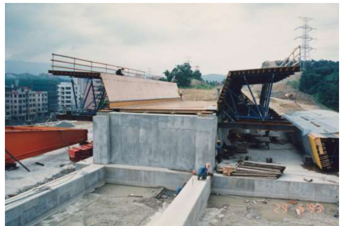
Typical ILM Deck Inner & Outer Form System
