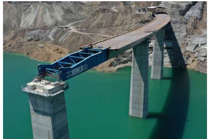
ILM Deck Launching
