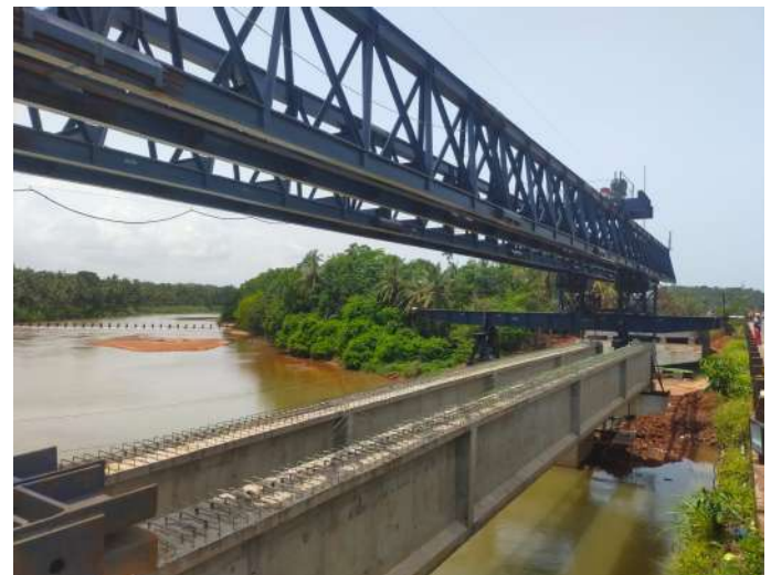
Section of Launching Gantry
