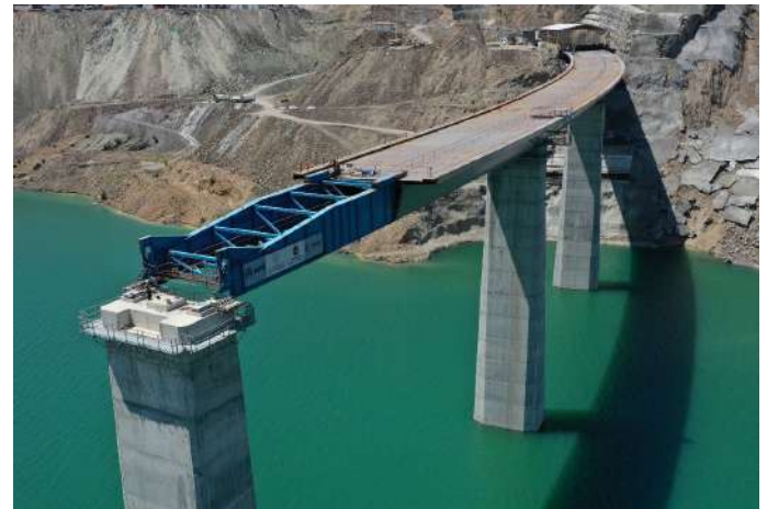
ILM Deck Launching
