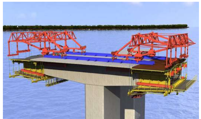
Typical FCC Deck Form Traveler
