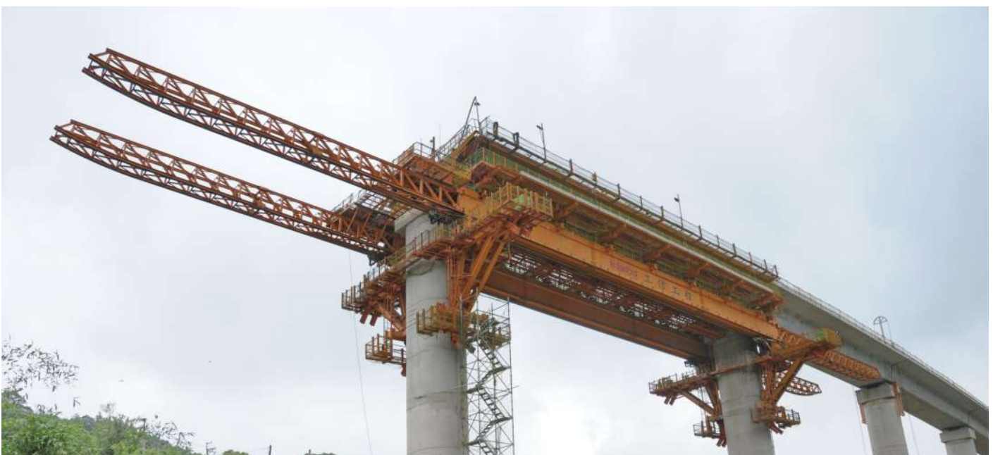
Typical Deck Inner Form System
