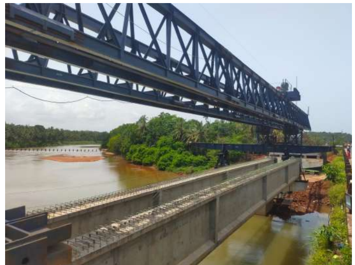
Section of Launching Gantry
